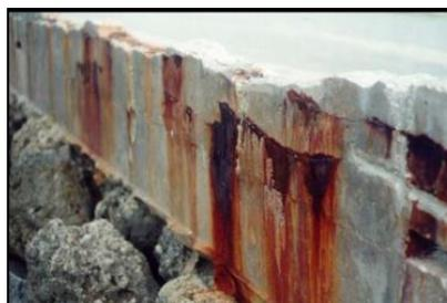
**Figure 1.3 :** Exemples: corrosion des armatures [5] [6]
