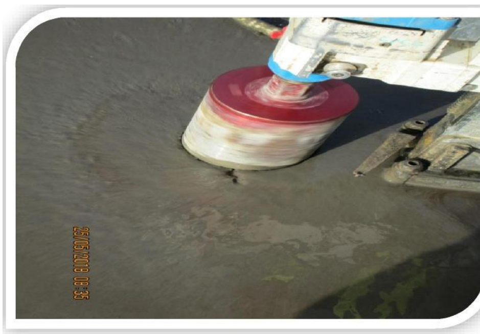
Figure IV .2 . Carotteuse
